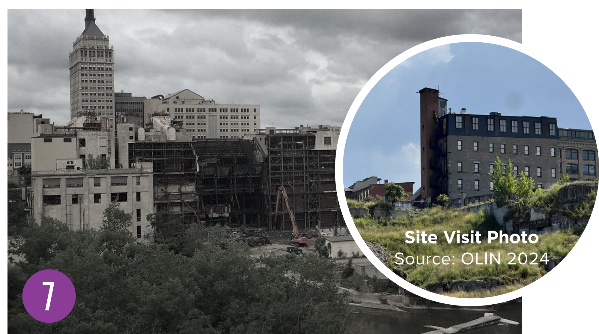
RG&E Beebee Station Demo, 2016 Source: The RochesterSubway
