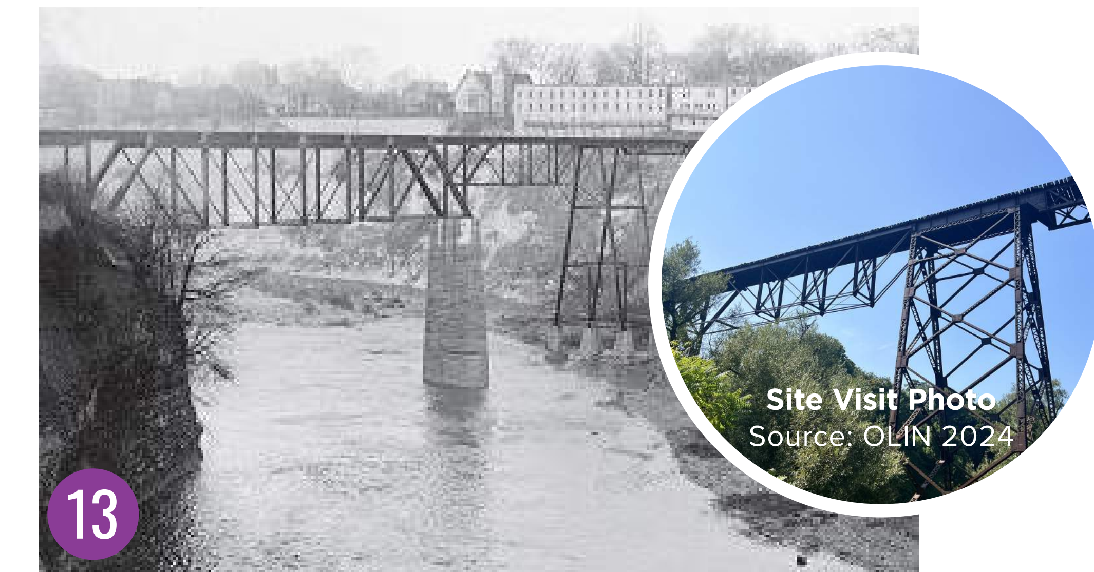
Running Track Bridge Source: Albert R. Stone Negative Collection, RMSC
