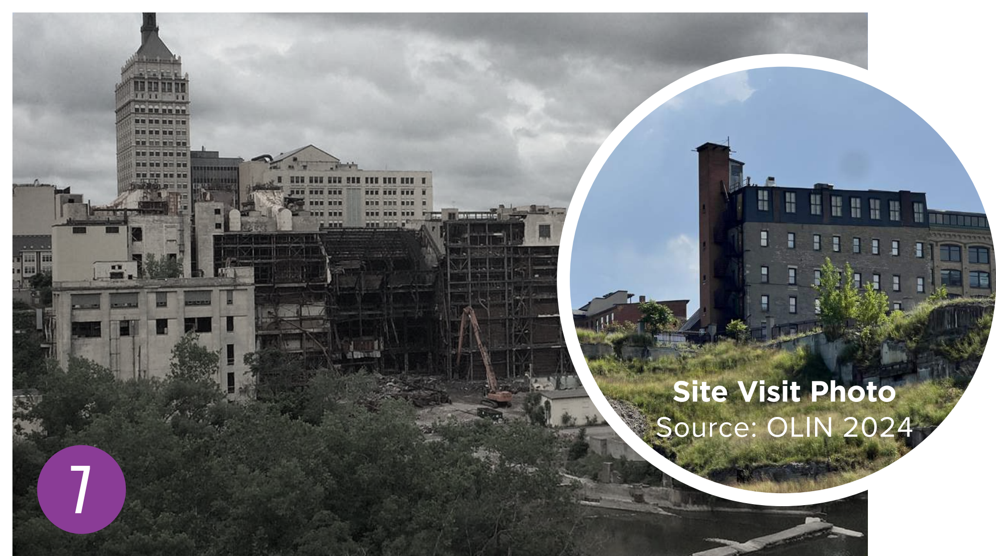
RG&E Beebee Station Demo, 2016 Source: The RochesterSubway
