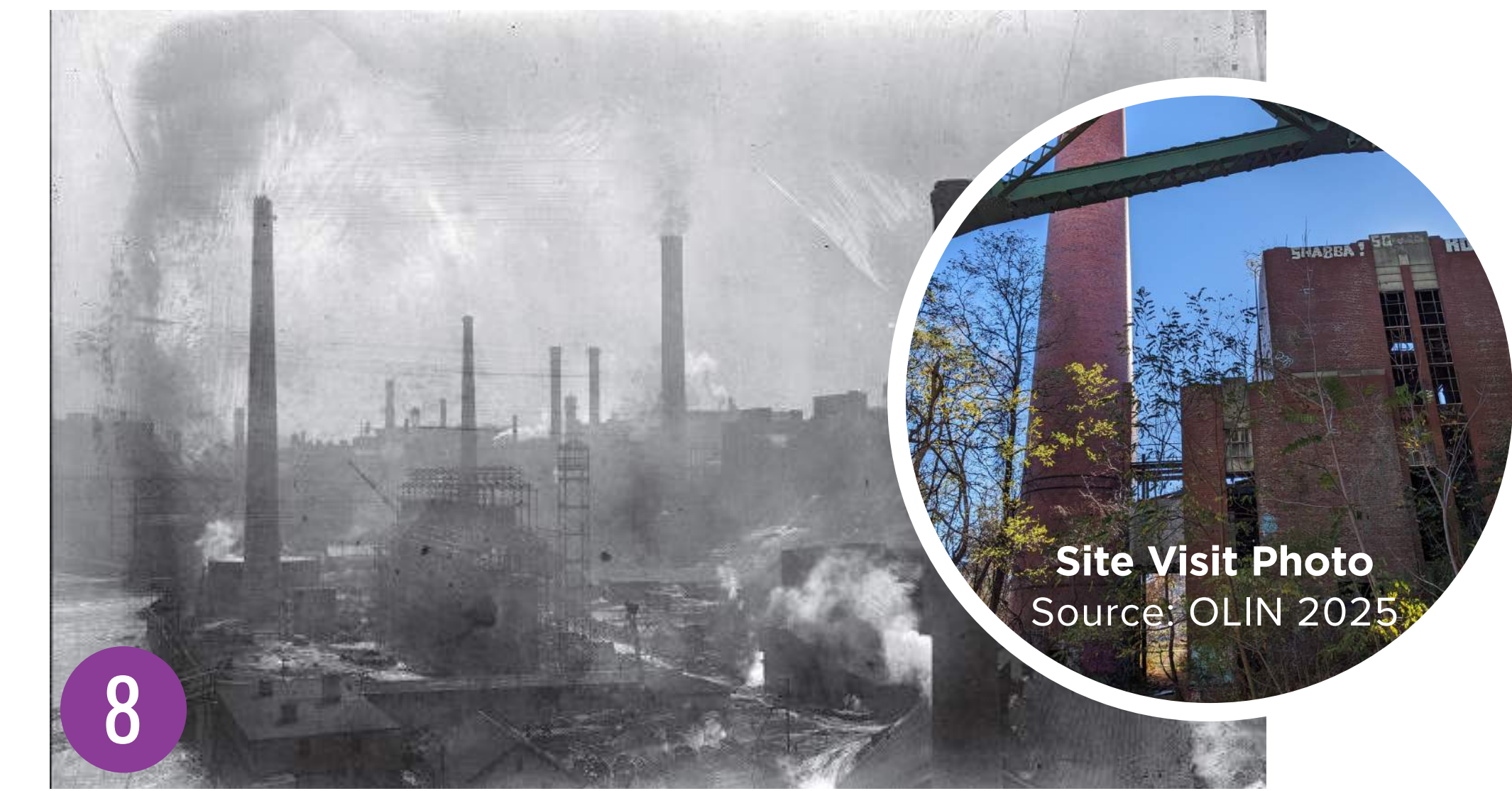
Incinerator And Coal Gasification Construction Looking Southeast, 1920s Source: Albert R. Stone Negative Collection, RMSC
