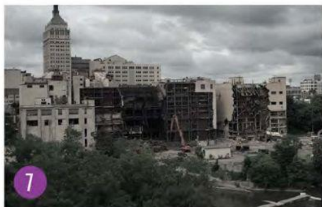
7 RG&E Beebee Station Demo, 2016 Source: The Rochester Subway
